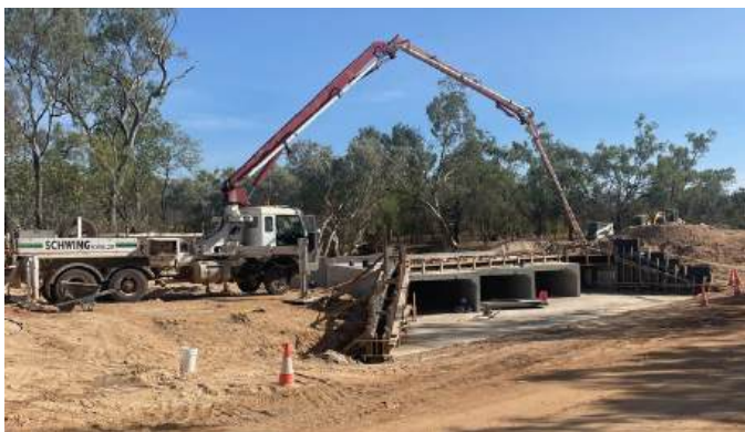
Base slab prep works.
