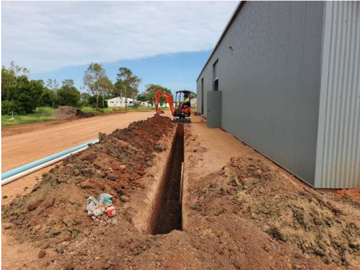
Photo: Plumbing works being installed at the new hatchery.
