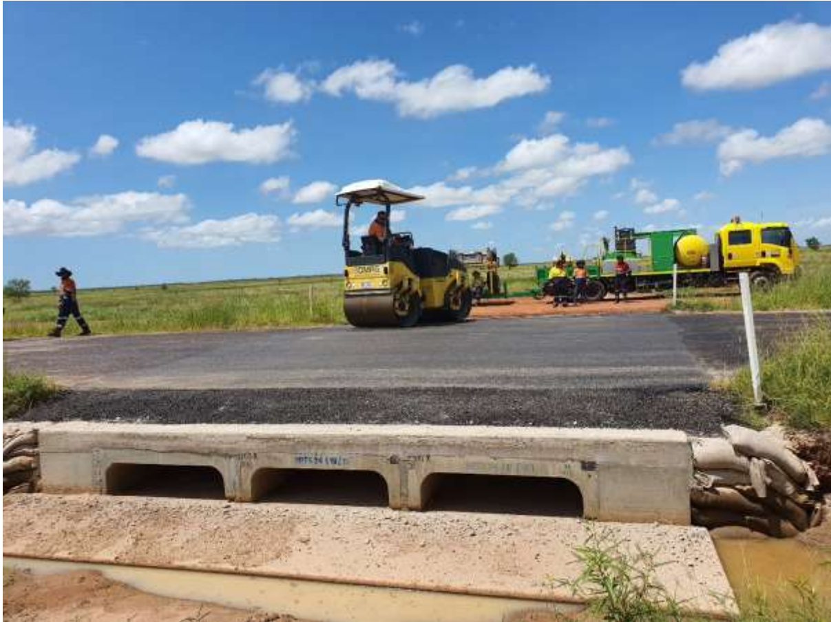
Photo: Asphaltting over the new culverts on the Karumba Road.
