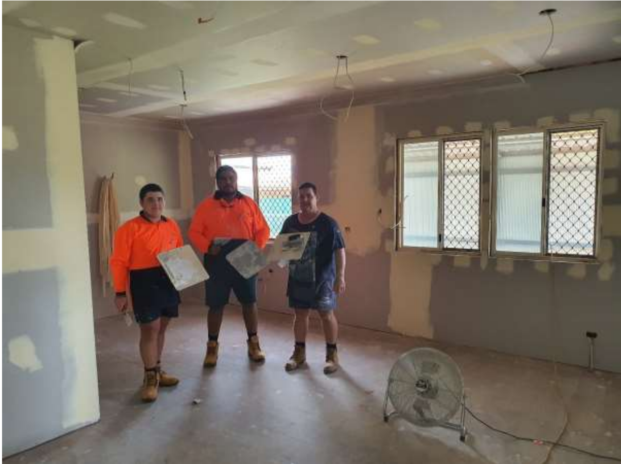
Photo: Work being done on 23 Woodward Street
