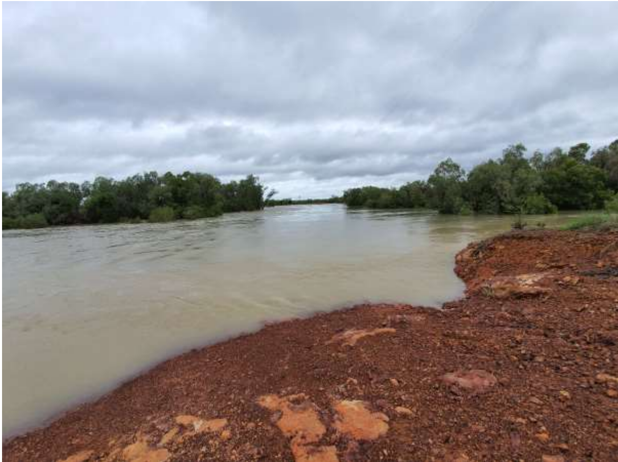
Photo: Glenore Weir under flooding 29 th January.
