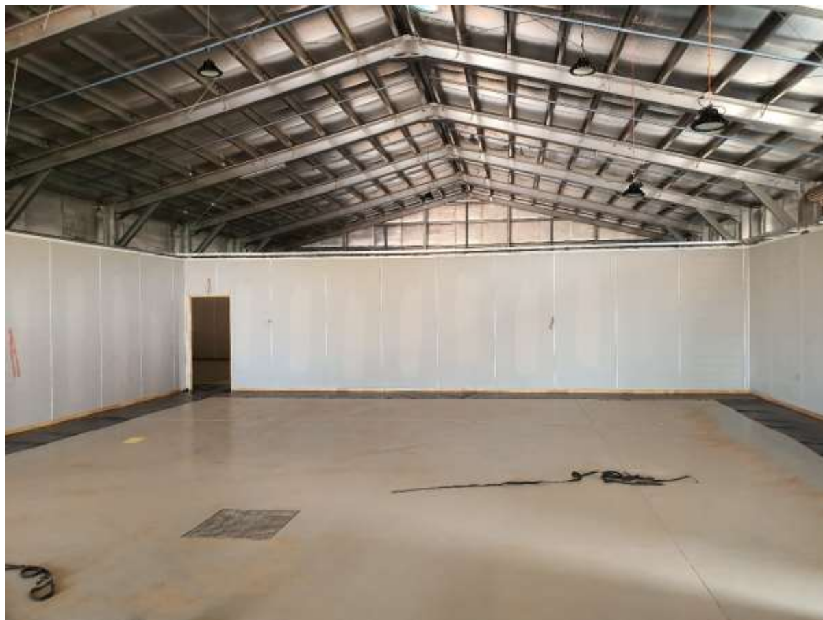
Photo: New Hatchery, internal painting underway.
