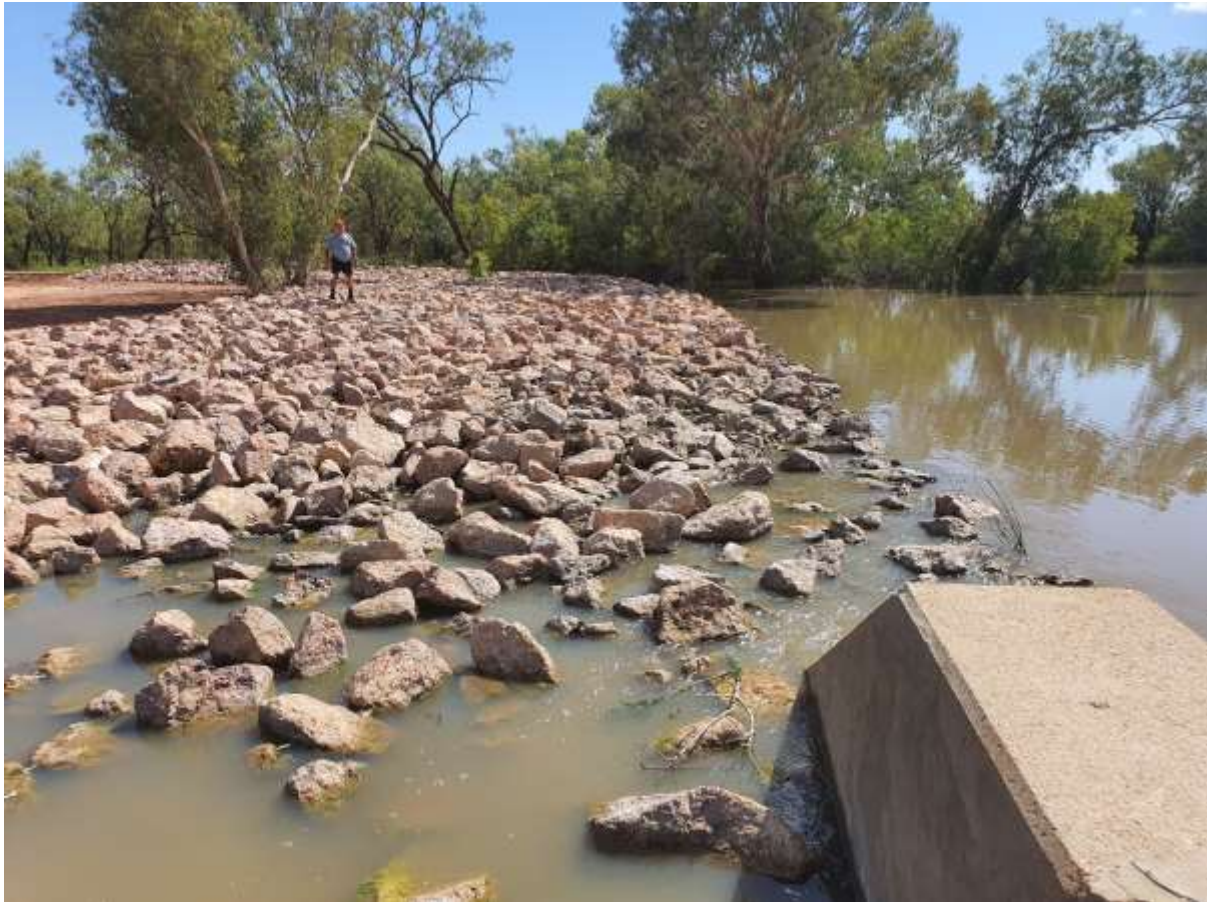
Photo: New rock work protection at Glenore Weir survived recent flooding.
