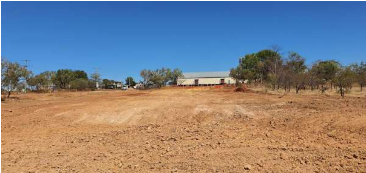
Photo: Excavation works on the Barge Ramp.
