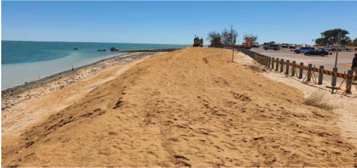
Photo: Sand replacement at Karumba Point.
