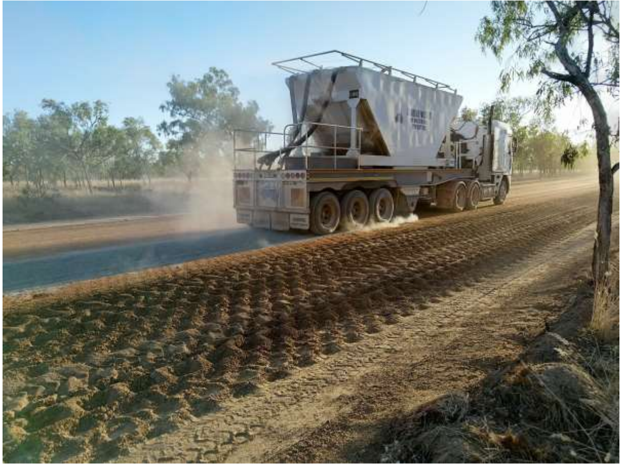
Photo: Spreader Truck spreading cement powder on road base on 89B.
