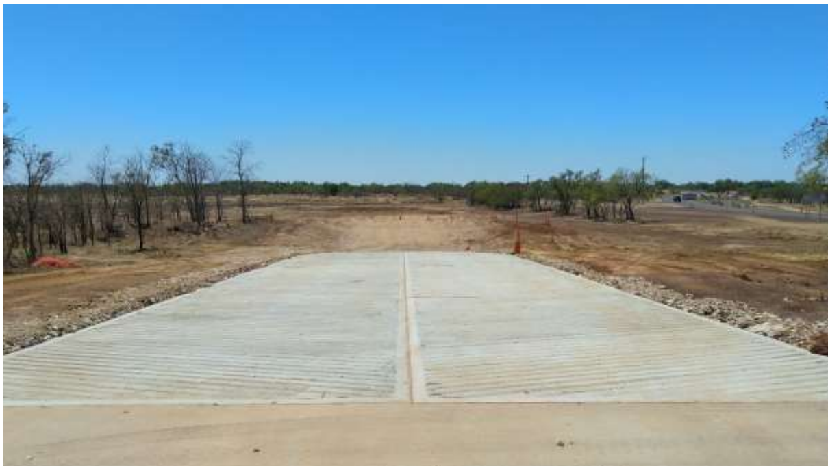
Photo: Completed Barge Ramp.
