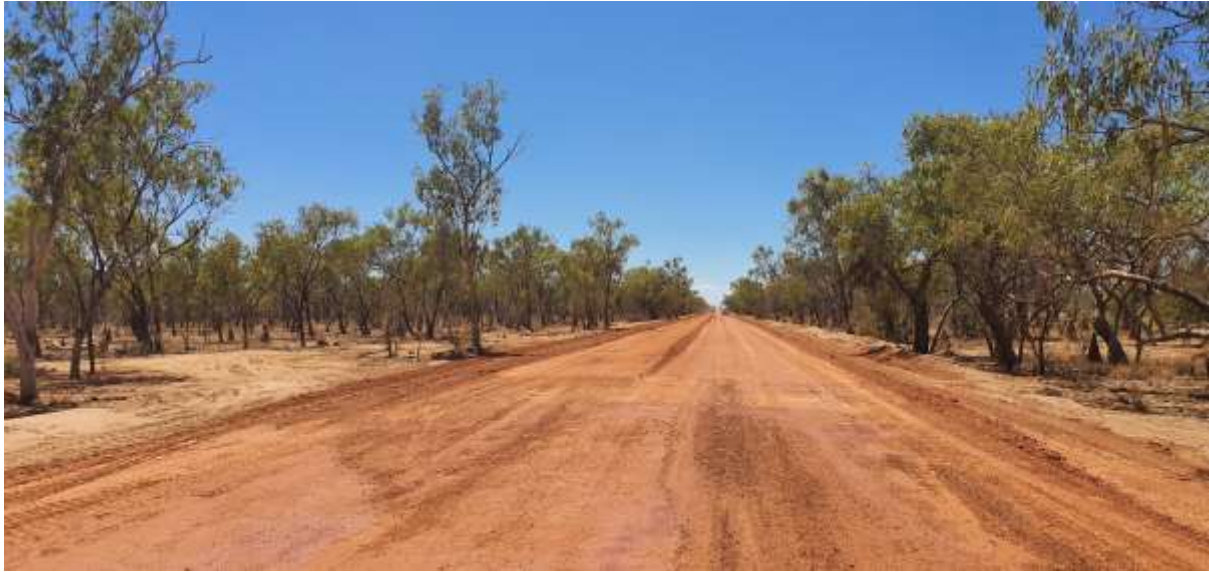
Photo: Preparing basecourse on 89B for the second 5km.
