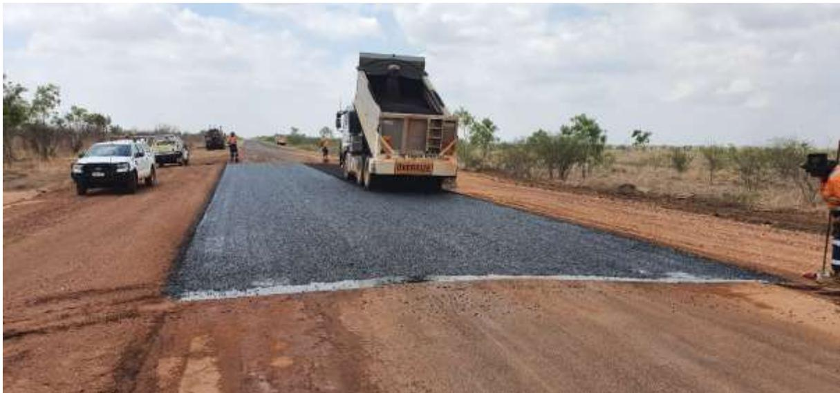
**Photo:** Sealing the repaired section where the dip was originally located on 89A.
