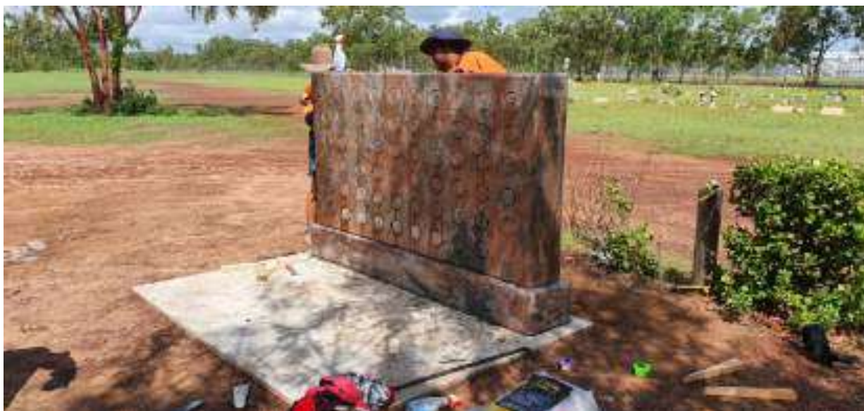
Photo: Completed Columbarium at the Normanton cemetery
