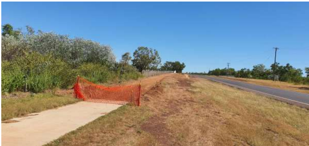
Photo: Excavation works have started for the footpath to the Rodeo
