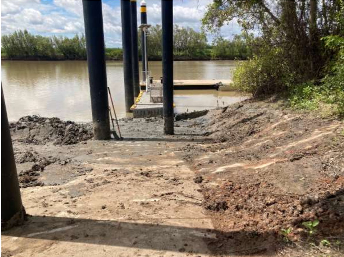
Photo: Cleaning up the Normanton Boat Ramp
