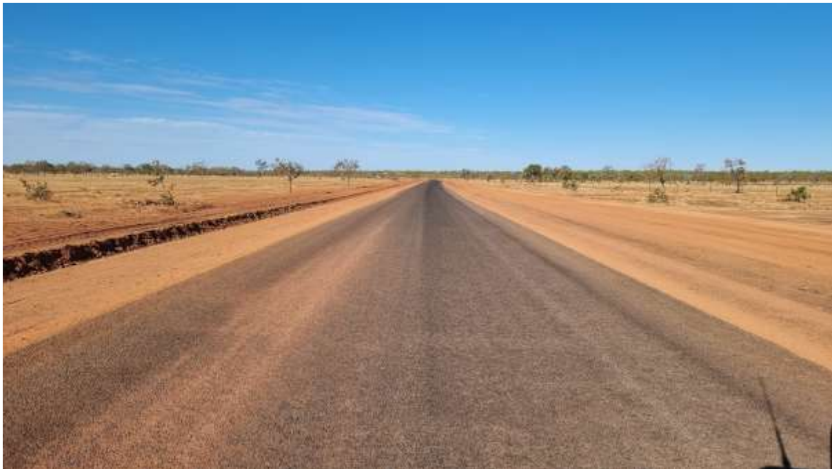
Photo: Burketown Road – TIDS work at Inverleigh
