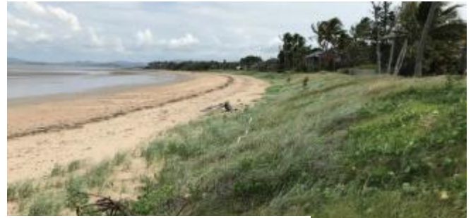
Buried geo-bag seawall at Zilzie, QLD
