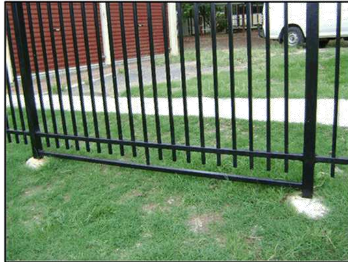
Picture 6.3: Type 1 Security Fencing with infill bar
