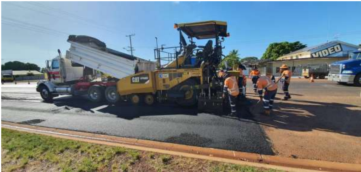
Photo: New Asphalt Works for the Pedestrian Refuge Crossing.
