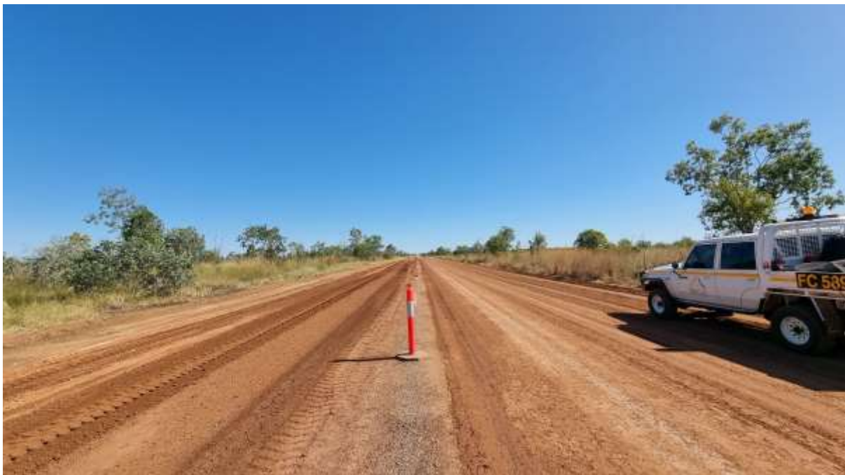
Photo: 89A – Rehabilitation Works (RMPC Variation)
