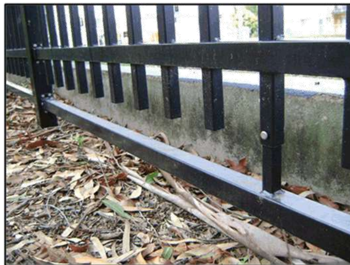
Picture 6.4: Type 1 Security Fencing with infill bar
