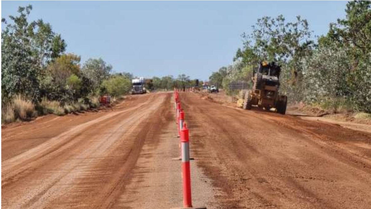
Photo: 89A – Rehabilitation Works (RMPC Variation)
