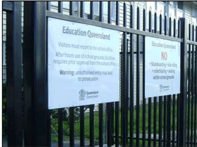
Picture 6.5: Signs correctly affixed to Type 1 Security Fencing
