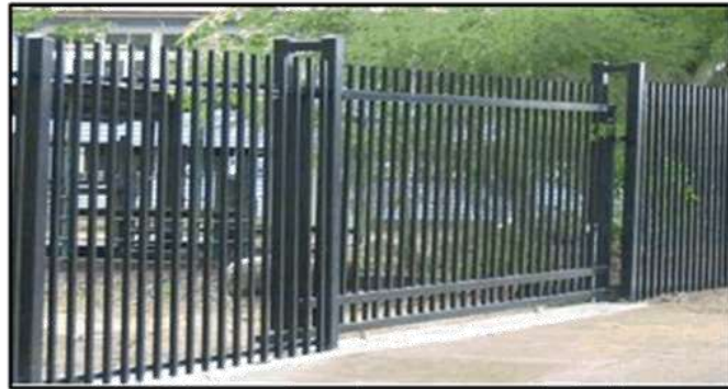
Picture 6.1: Type 1 Security Fencing Sliding Gate
