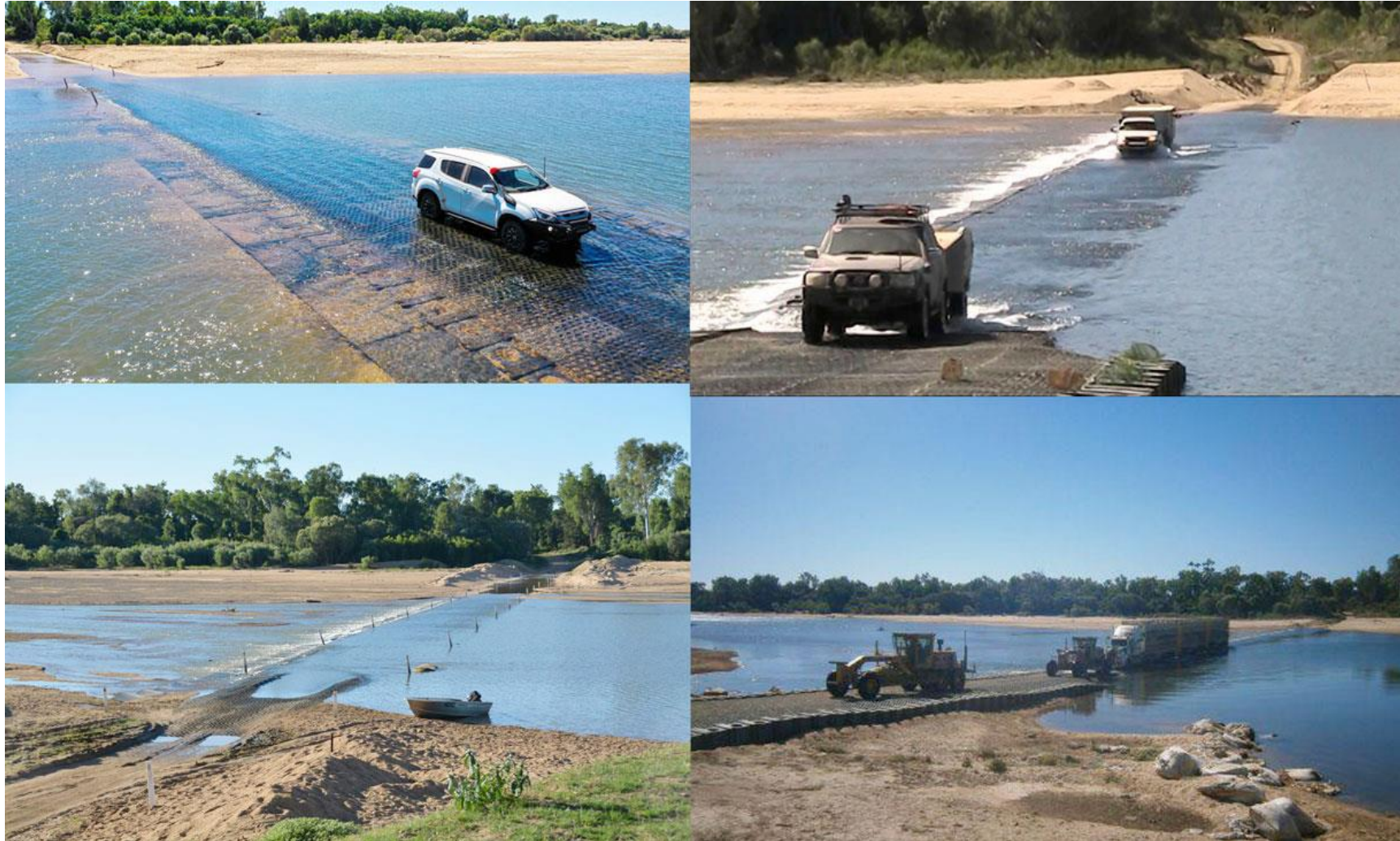
Photo 4 - Dunbar Crossing of the Mitchell River
