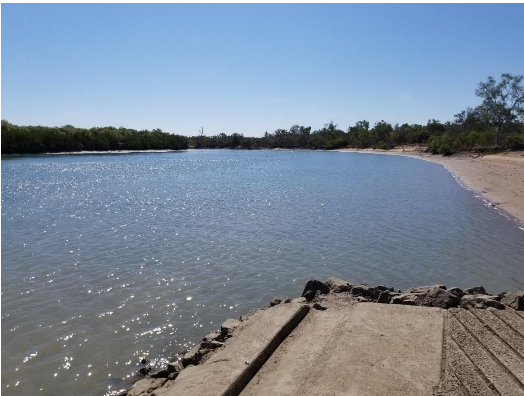
Photo 13 - Barge Ramp Topsy Creek, Kowanyama
