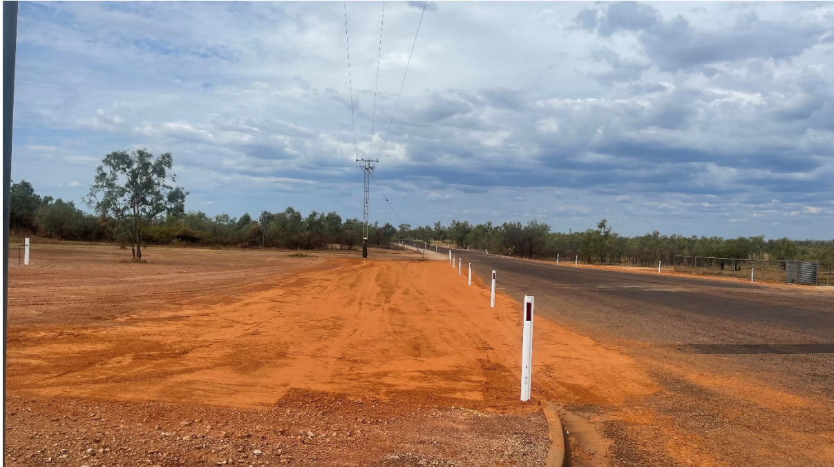
Photo: Thompson Street Kerb and Channel – Completed Earthworks
