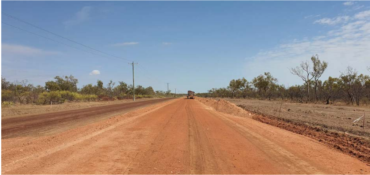
Photo: Lilyvale Subdivision – Internal Roadwork
