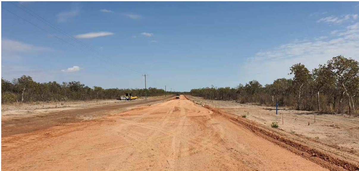
Photo: Lilyvale Subdivision – Internal Roadwork
