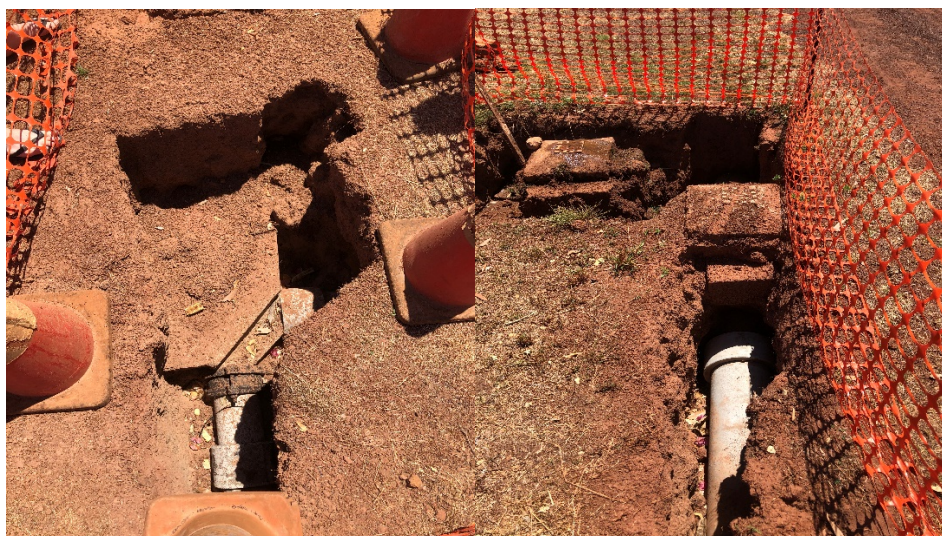
Figure 9: Merge of Raw Water Mains
