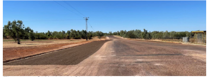
Thompson St Kerb and Channel project sealed.
