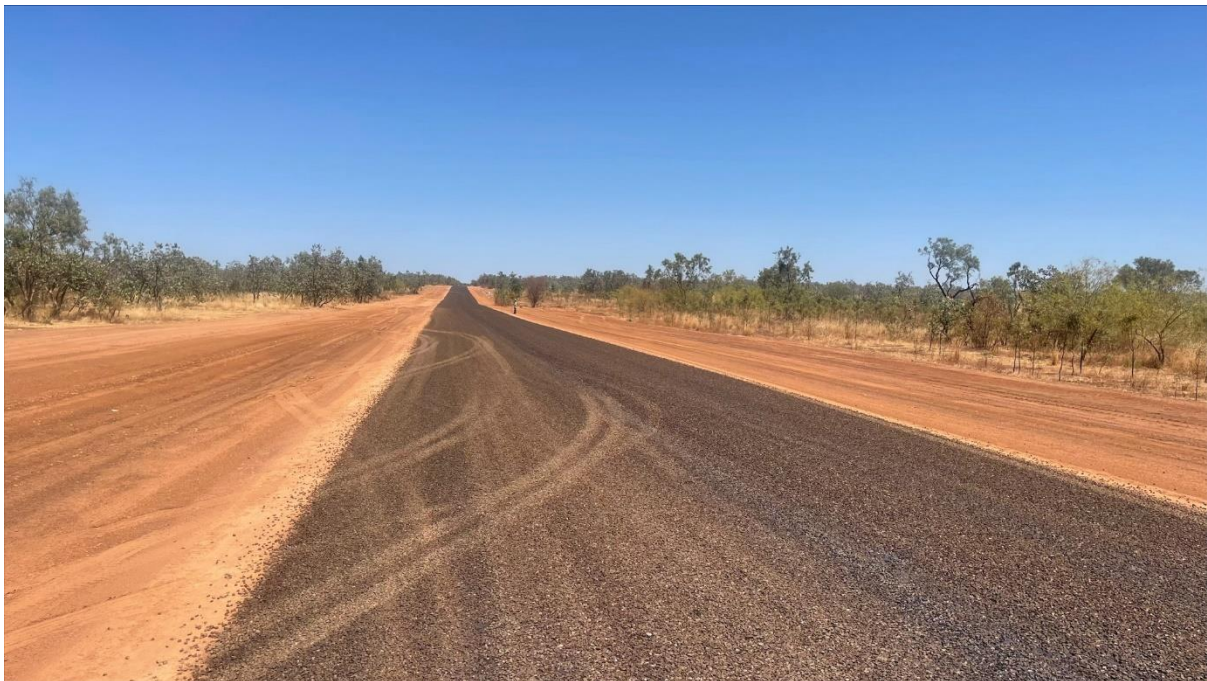
Photo: Shoulder reconstruction work on 89A
