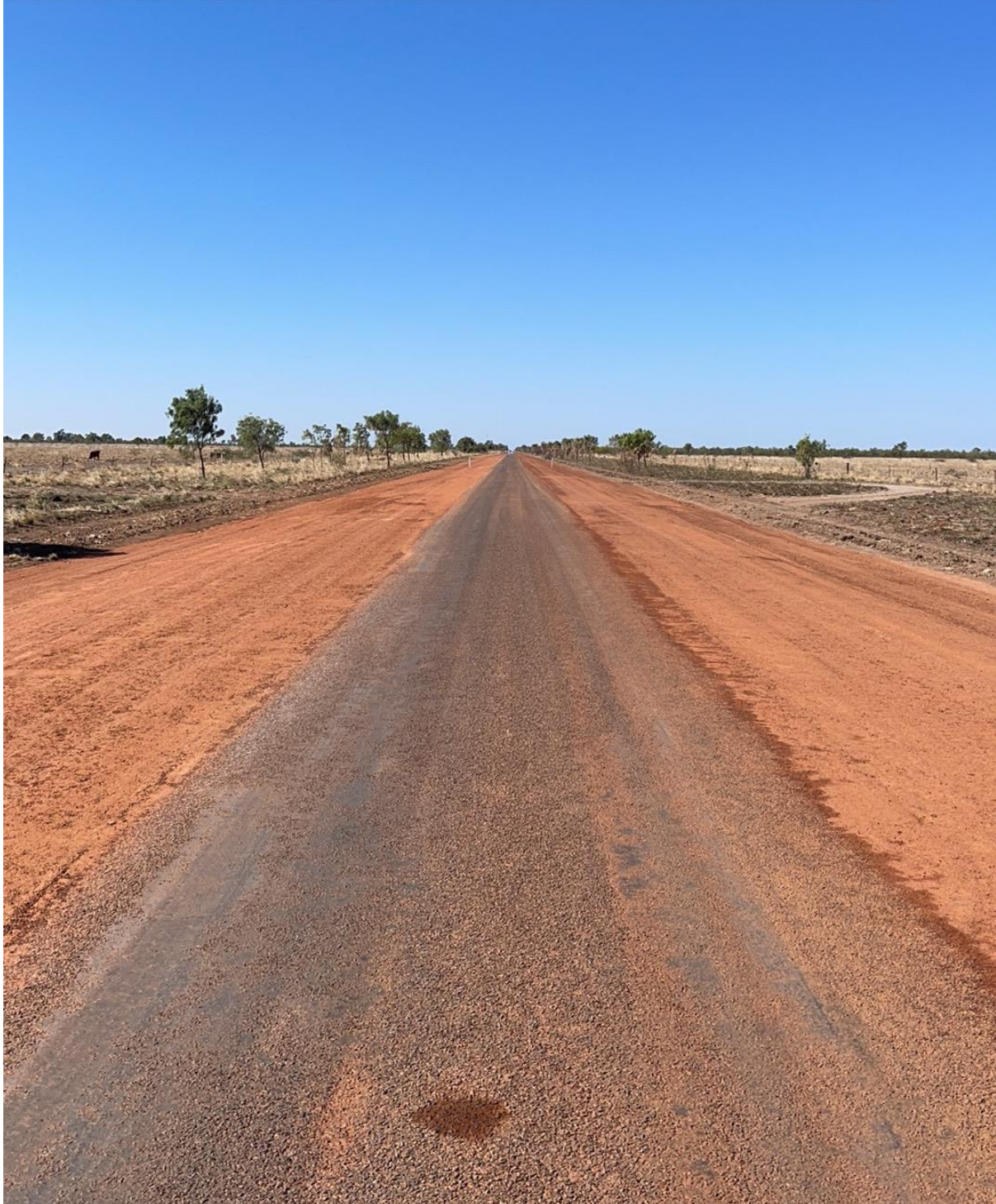
Photo: Shoulder reconstruction work on 89A
