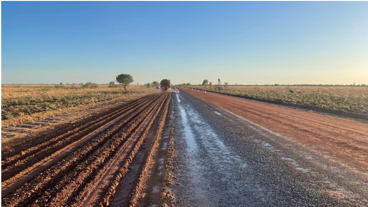
Photo: Normanton - Burketown Road 3km sealing TIDs project
