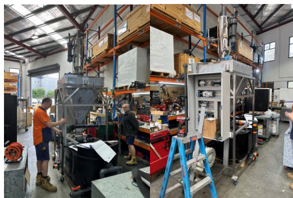
Figure 7 - Soda Ash Dosing System Construction Progress
