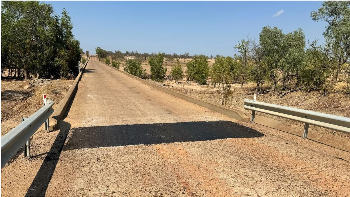
Photo: Premix repair at the Flinders River – Normanton Burketown Road
