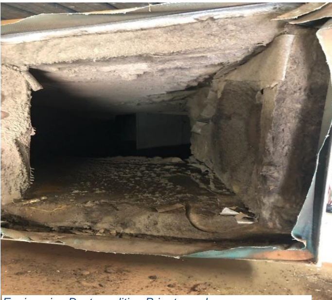
Engineering Duct condition Prior to works
