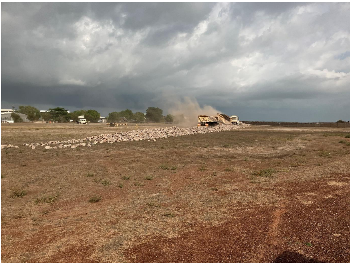
Photo: Revetment Wall rock being delivered to Karumba
