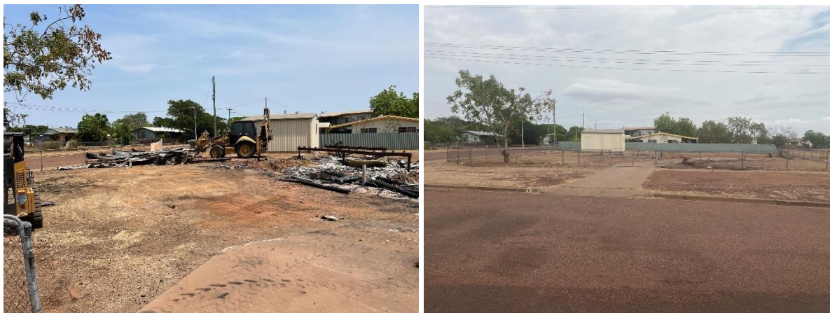
Figure 3 – 17 Palmer Street – Clean up in Progress.
