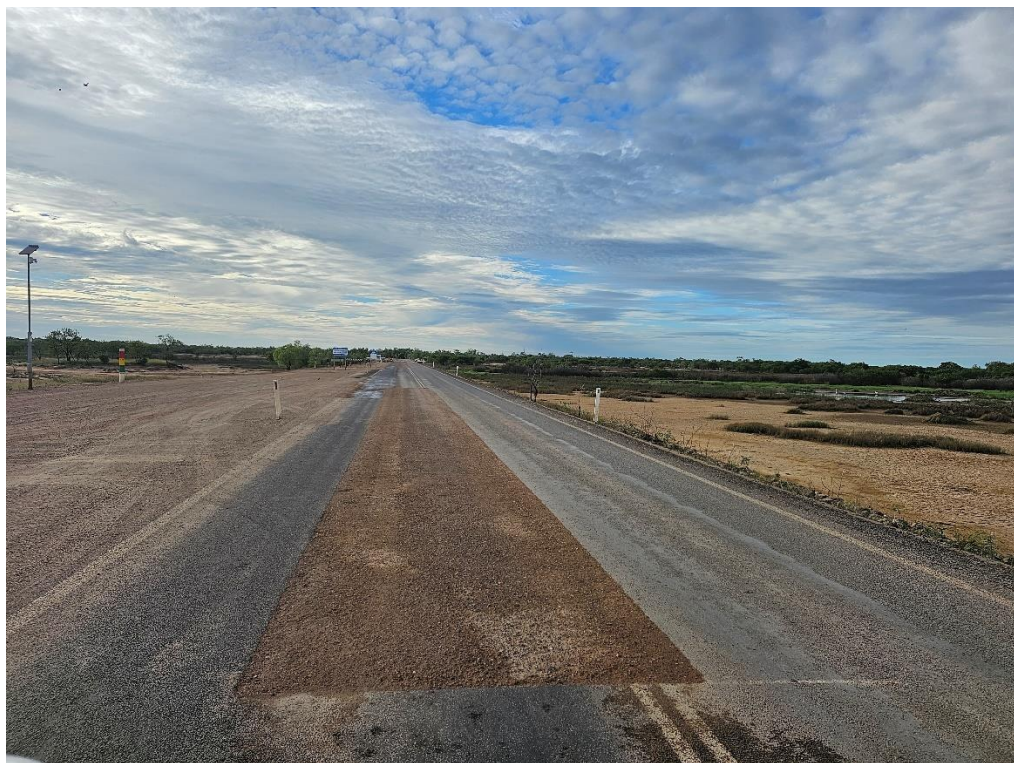
Photo: Stabilised repairs and shoulder works before Corduroy
