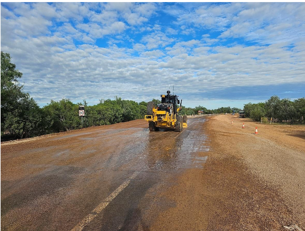
Photo: Stabilised repairs and shoulder works after Corduroy
