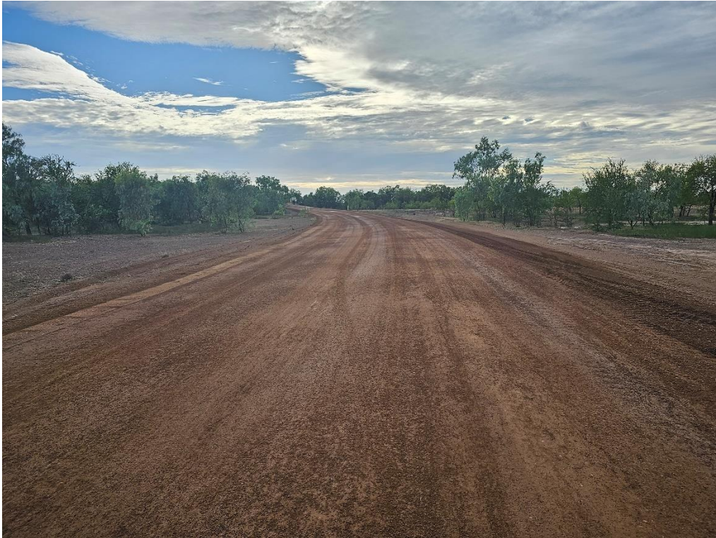
Photo: Stabilised repairs - Norman River Foot Bridge
