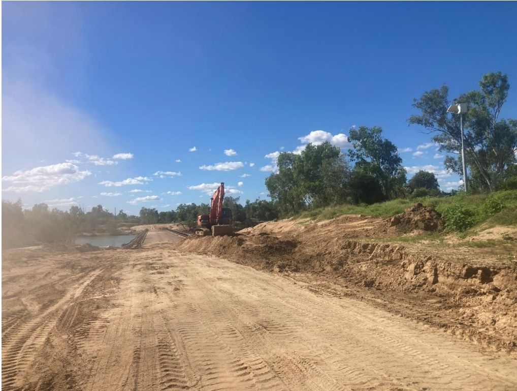
Photo: Sand being removed from the Gilbert R on 89B
