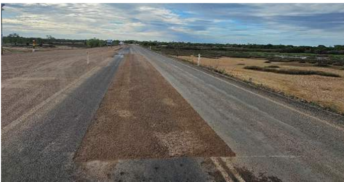
Stabilised repairs and shoulder works before Corduroy
