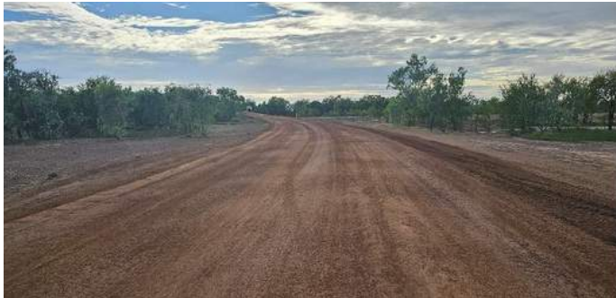
Stabilised repairs - Norman River Foot Bridge
