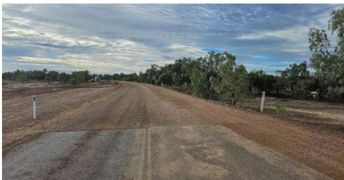
Stabilised repairs and shoulder works after Corduroy
