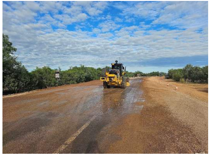
Stabilised repairs and shoulder works after Corduroy
