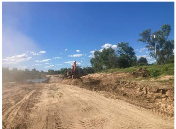
Sand being removed from the Gilbert R on 89B
