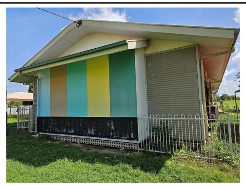
Photo: Northern Wall using Fibre Cement Sheets.
