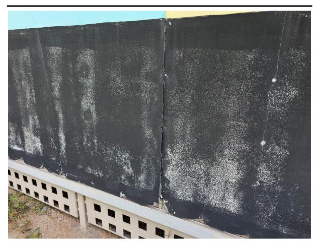
**Photo:** No sealant at the joint causing moisture ingress and minor lifting at the edge.
