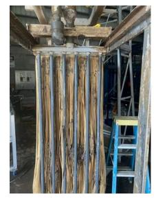
Photo: Membrane De-ragging and inspection
