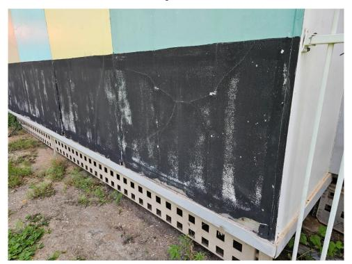
Photo: Faded Paint, unpainted edge resting on lip causing moisture ingress.
