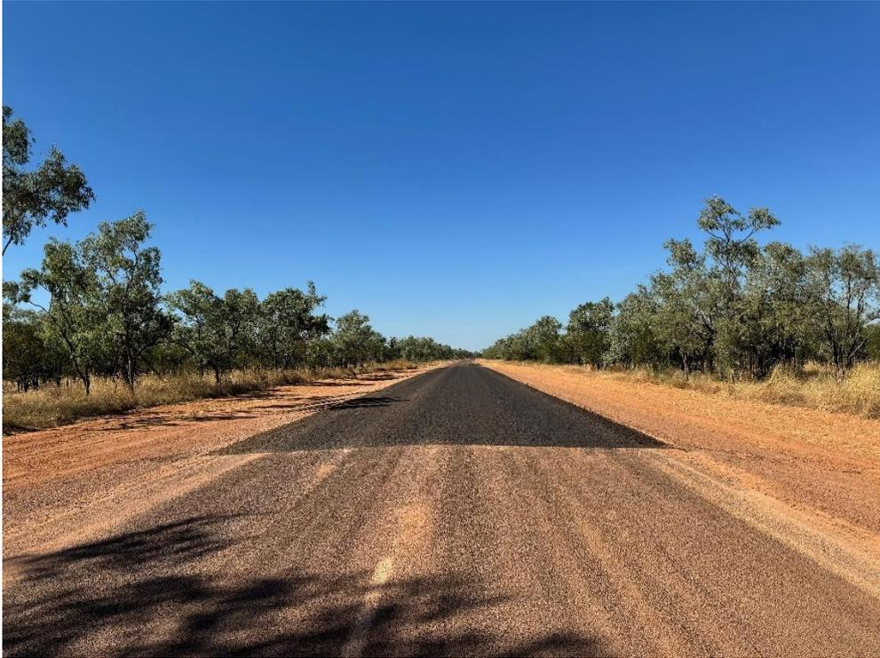
**Photo:** Patch repairs on 92A Croydon Road
