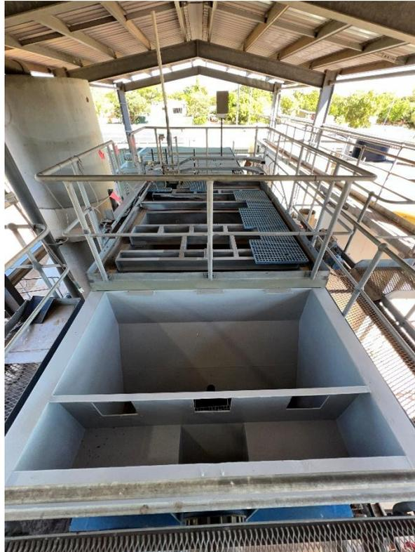
**Photo:** Normanton WTP Clarifier No.1 Sand Blast and Re-Coat
