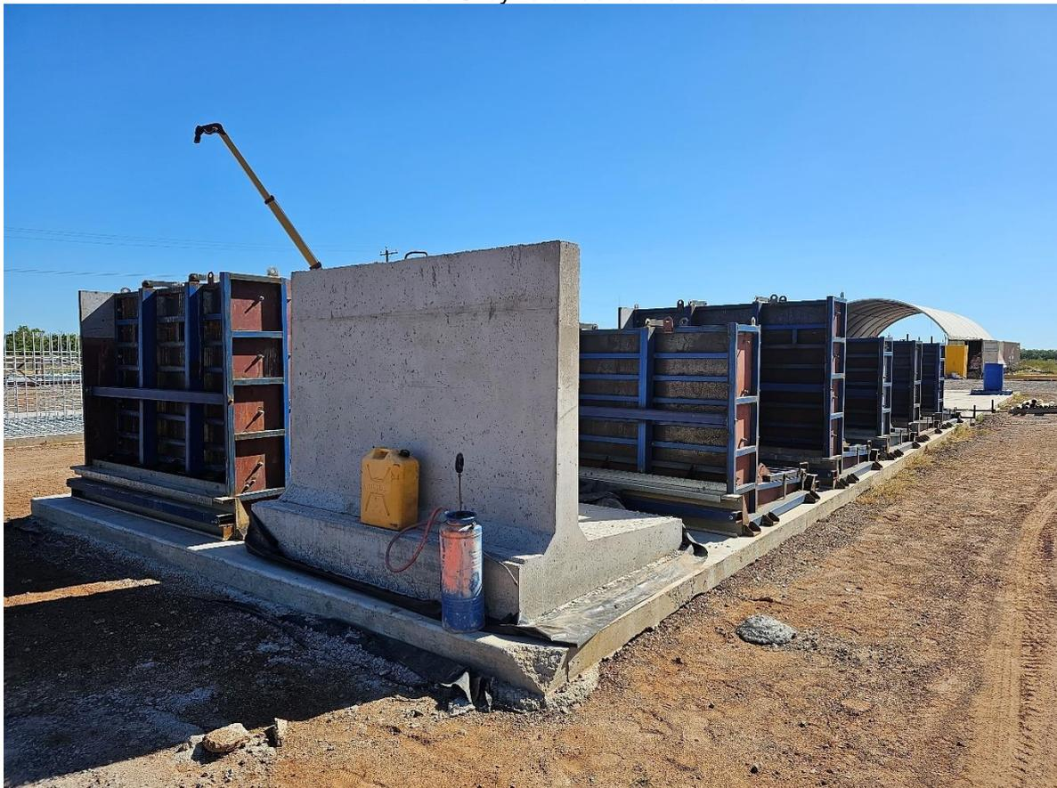
**Photo:** Precast walls for the Revetment Wall under construction
