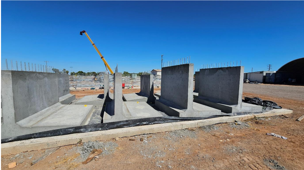
Photo: Precast walls for the Revetment Wall under construction
